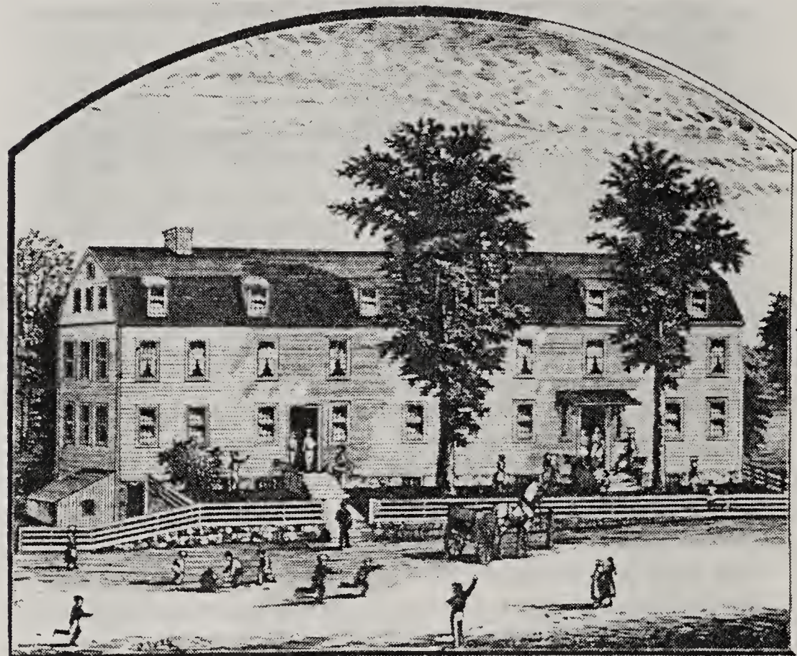
NINE PARTNERS BOARDING SCHOOL
